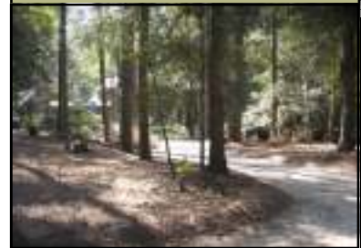
A sinking road
